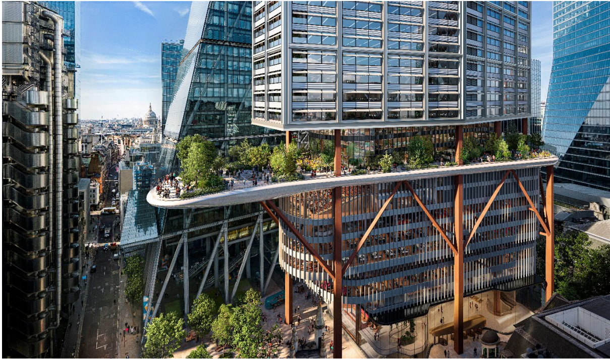
Level 11: a free-to-access elevated public podium garden © One London
